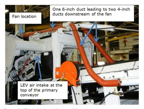
Figure 6: LEV air intake at the top of the primary conveyor.
