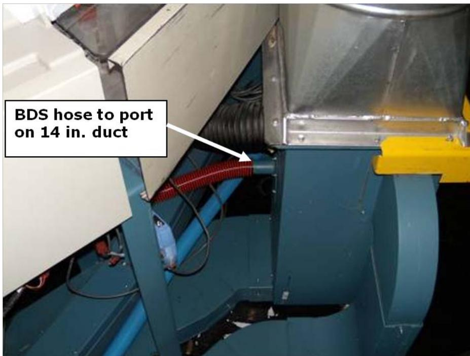
**Figure 21: BDS hose (in orange) routed to a port near the base of the 14 in. VFS duct**
