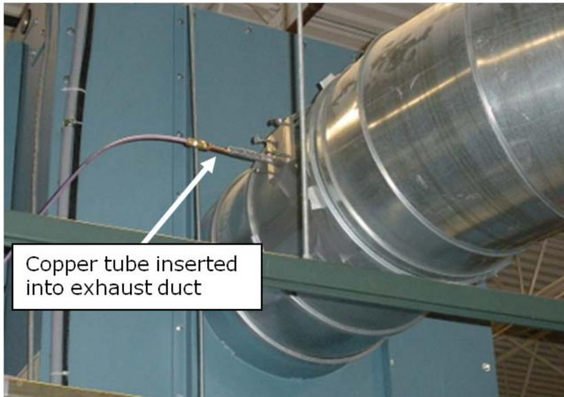
**Figure 4: Copper tube to sample tracer gas from exhaust duct**
