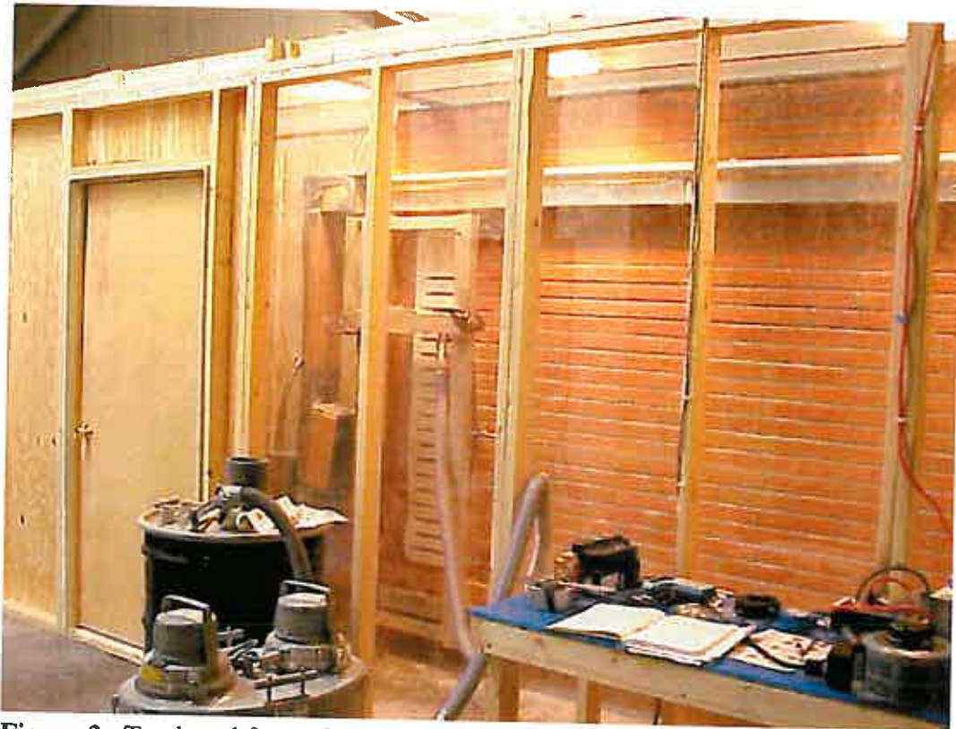
Figure 3. Track and frame for mounting and moving the tool down the wall.
