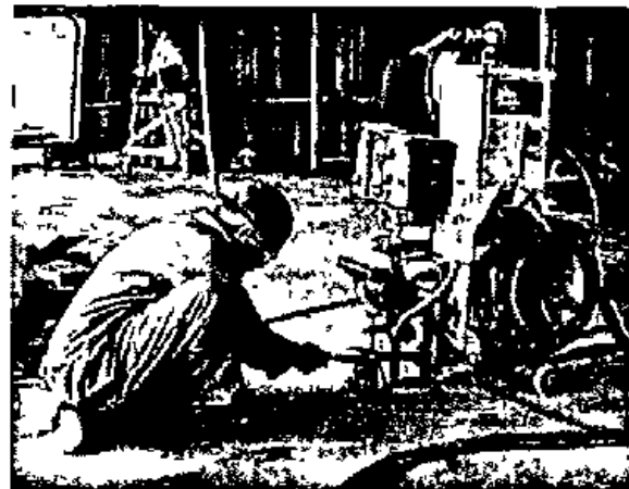
Figure 8 Worker operating semi-automatic wire-feed welder
