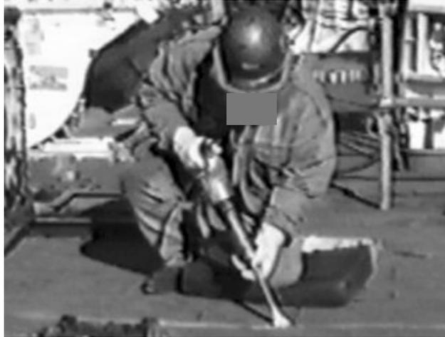
Figure 8. Worker Using Chipping Hammer to Remove Terrazzo Tile from Deck Surface
