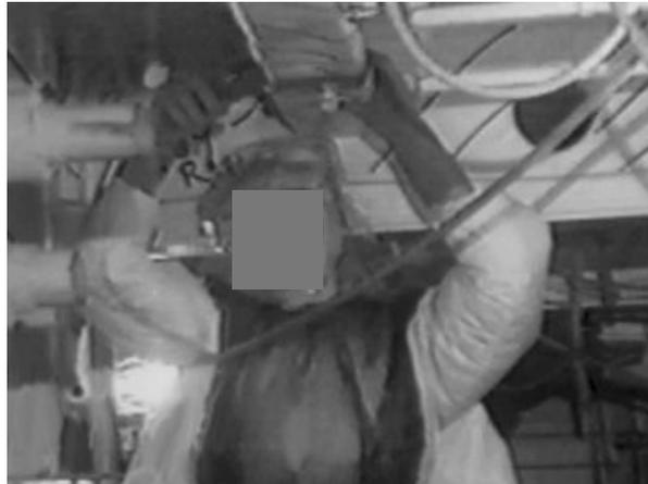
Figure 4. Insulation Worker Cutting into Insulation with Hawkbill Knife
