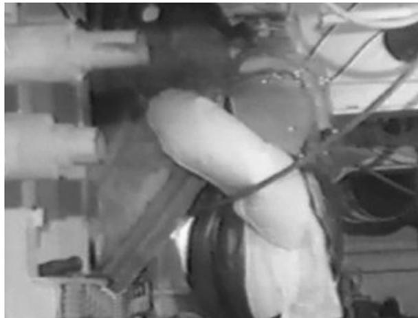
Figure 5. Pulling Section of Insulation Off Bulkhead by Hand
