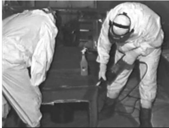
Figure 6. Two-Person Cutting Operation for Ductwork with Possible Hazardous Material
