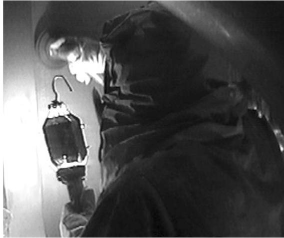
Figure 15. Tank Grinder Using 5-Inch Offset Grinder
