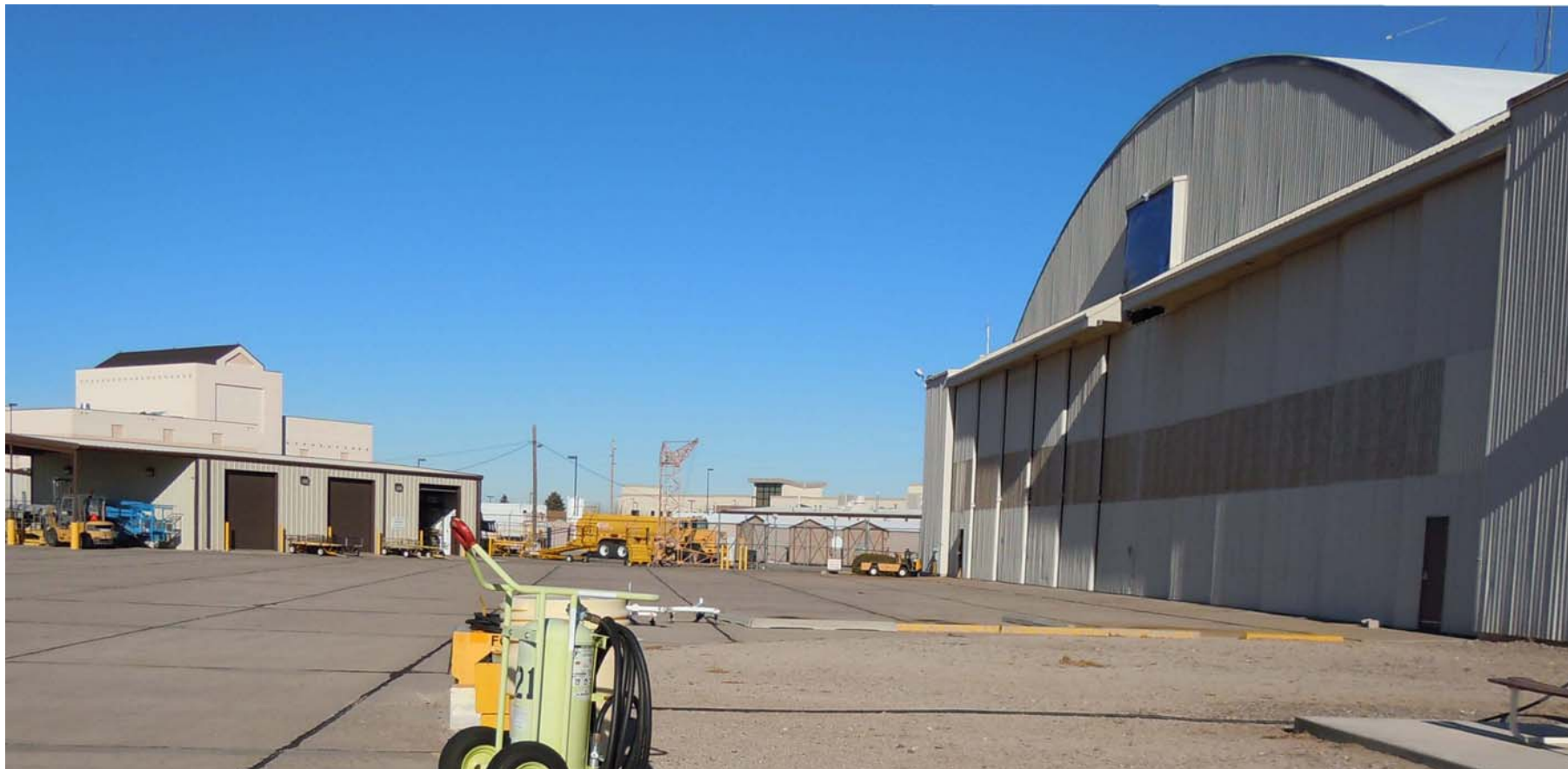
Figure 5-4: Photo of Hangar 481 and Associated Shop Buildings
