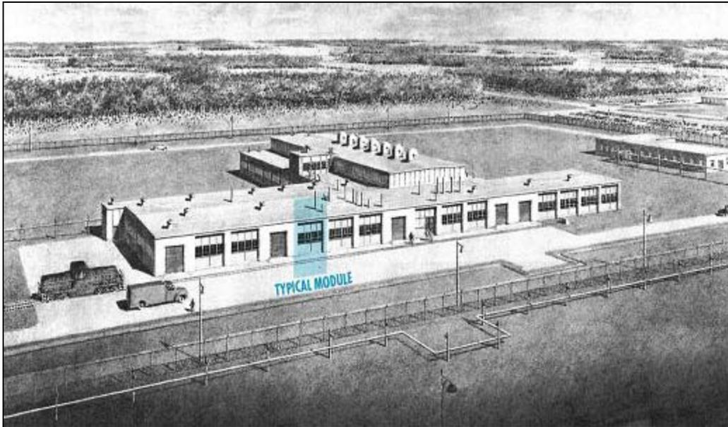
Figure 1. Architectural sketch of Building 313-M emphasizing the modular design of the facility. The east side of the building is facing the viewer.
