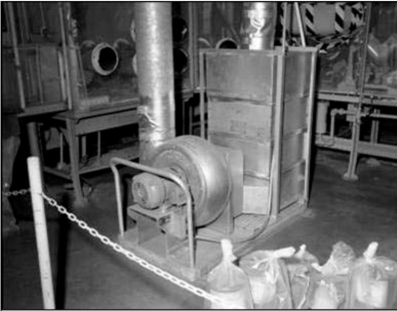
Figure 9. HEPA filter and ventilation blower for the enclosure. Also note the bagged cans of material in foreground behind the radiological chain. Source: Coughenour (2009). The photograph is unclassified and does not contain UCNI.
