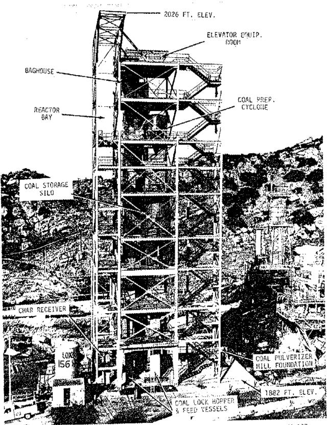
Figure 2. 3/4 TPM Hydrogasification IPOU Facility: Construction Progress on December 31, 1980
