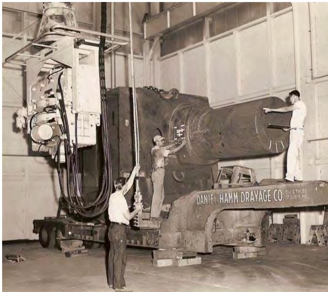
Figure 3. Betatron Radiography of the Axle of a Power Shovel Cast at GSI
