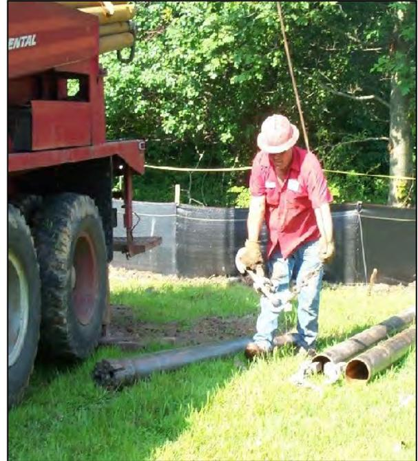
**Case 2:** A crew was preparing to remove a pump from a well when the hoist boom contacted a 4160-volt power line. The hoist operator was electrocuted.
