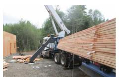
**Figure 3.** Truck-mounted crane with trusses on the trailer
