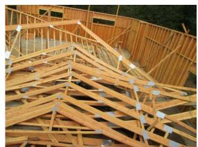
**Figure 1.** Collapsed trusses where the incident occurred.
