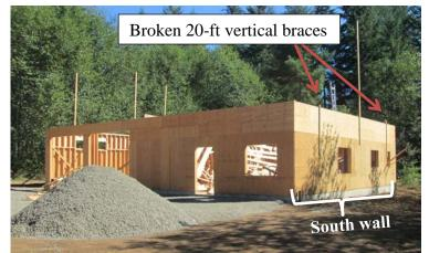
**Figure 2**. The shop/garage building with collapsed trusses within the structure. Note the 2X4's nailed to the outside of the south wall and that ground bracing was not erected. Middle vertical brace remained unbroken.
