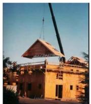
Example 1. Erecting and sheeting a series of trusses on the ground and then lifting the unit into place with a crane.
