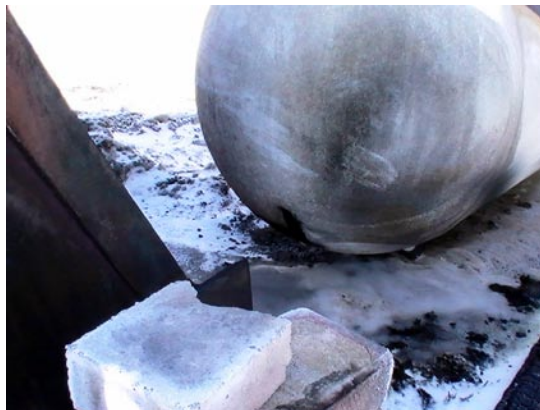
Figure 4. Damaged propane tank and the final location of loader bucket.
