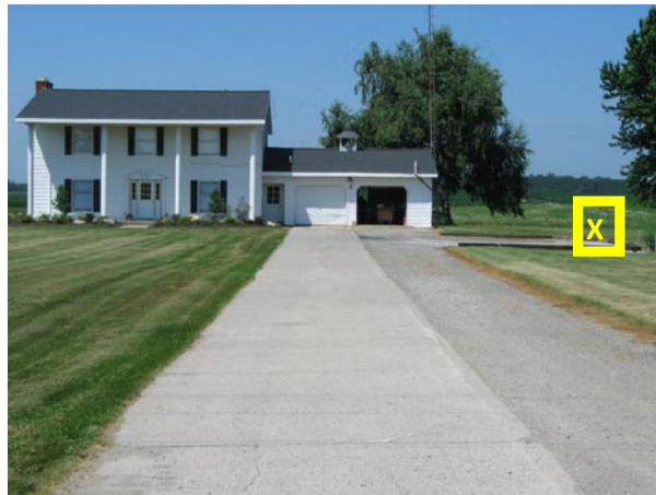
Figure 2. Driveway and turnaround leading to house. X signifies propane tank location.
