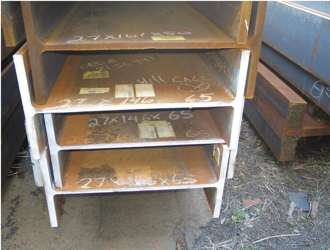
FIGURE 5. Stable, centered stack of steel beams.
