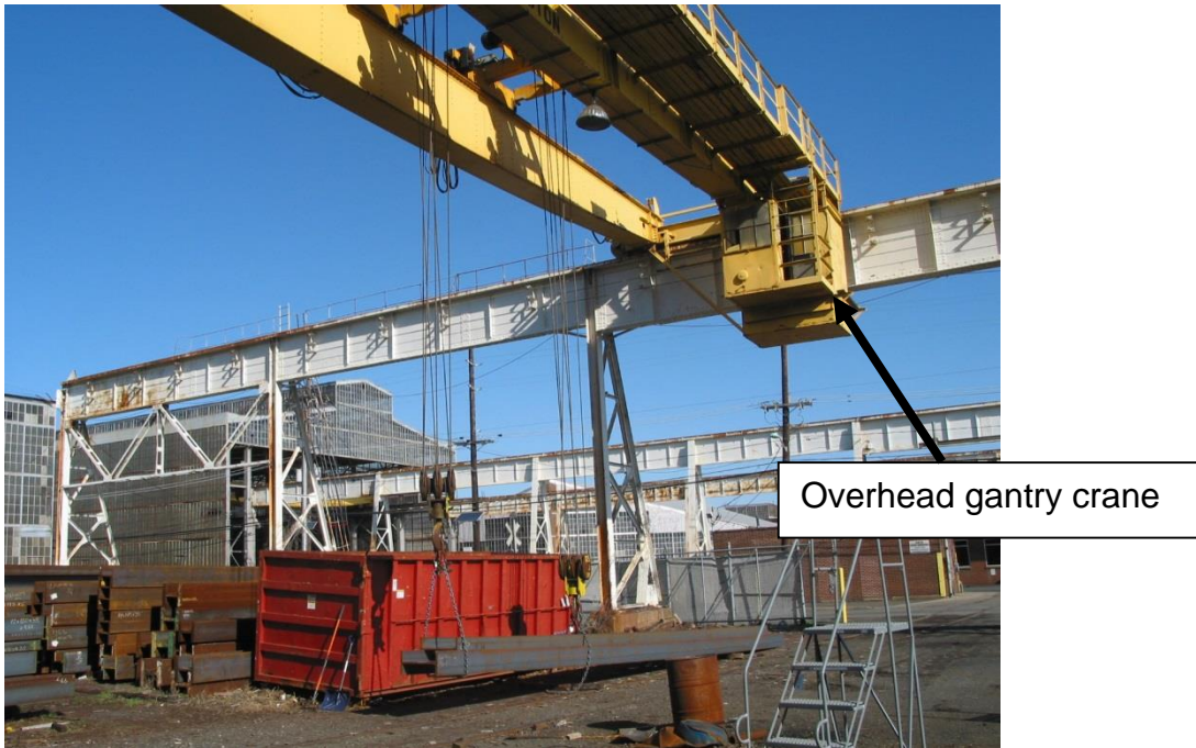
FIGURE 1. Incident site, the yard of a steel beam warehousing facility: a) gantry crane; b) stacked beams.
