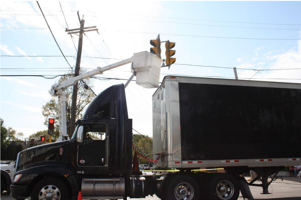
Figure 4 – Tractor-trailer with raised bucket
