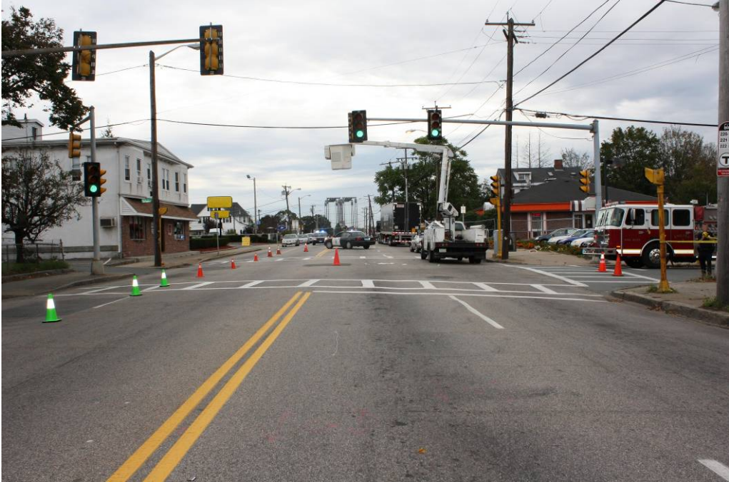
Figure 3 – Incident location with vehicle-mounted aerial lift
