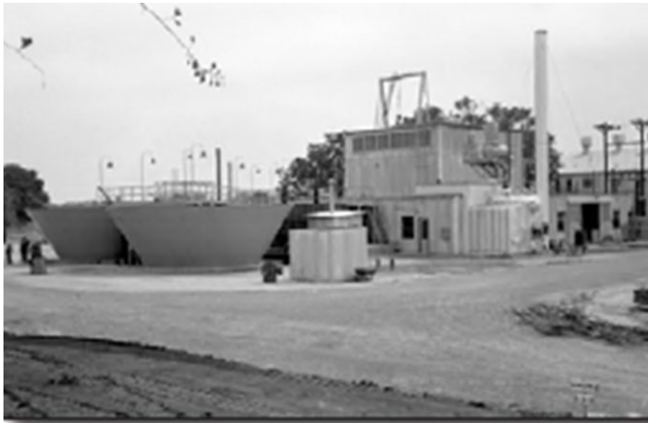
Figure 2-38. CMX Building 679-T [Swanson and Reed 2006, p. 68].
