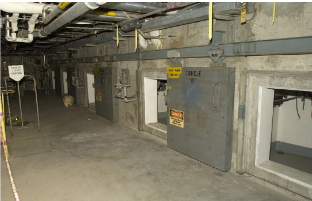
Figure 2-12. View of Purification Area cells [Reed 2010, p. 183].
