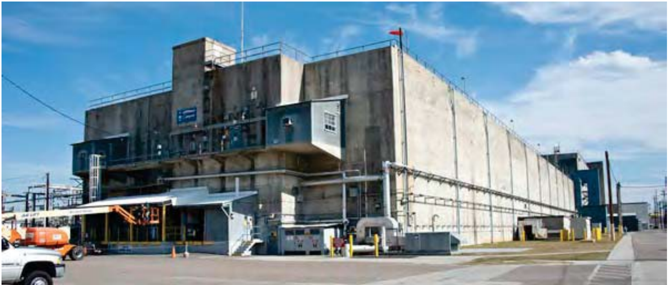
Figure 2-23. 221-H Canyon building [Reed et al. 2013, p. 23].
