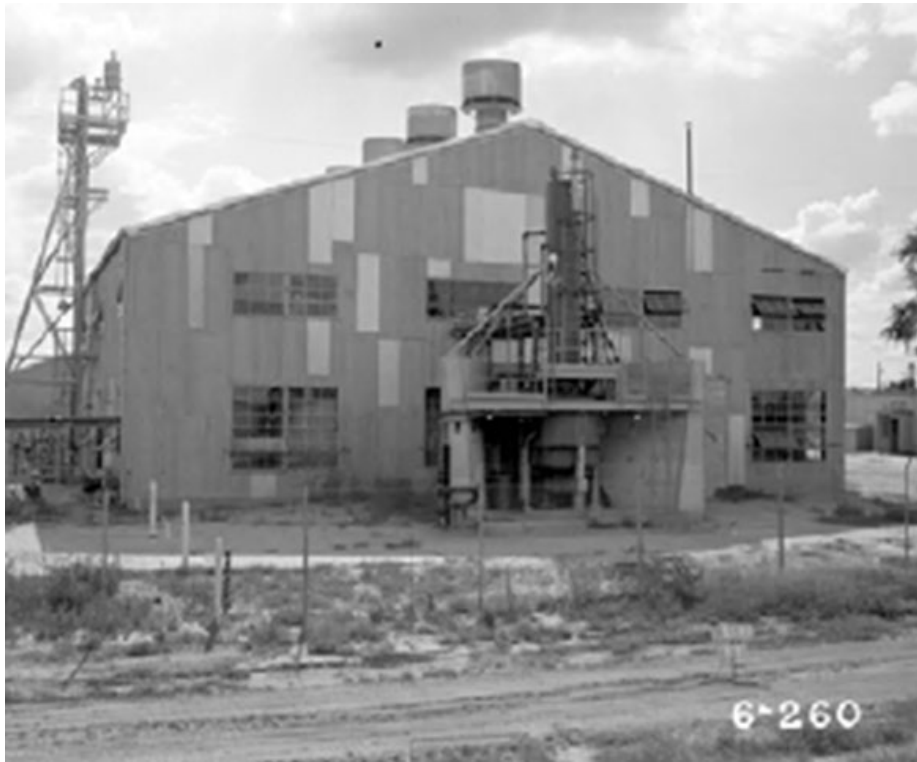
Figure 2-39. TNX Building 678-T [Swanson and Reed 2006, p. 74].
