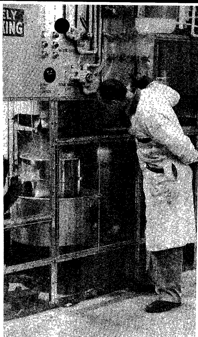
AGGLOMERATION, or "gathering together," of UO_2 powder, starts the pelleting. Checking is Jan Ericson, chemical engineer.
