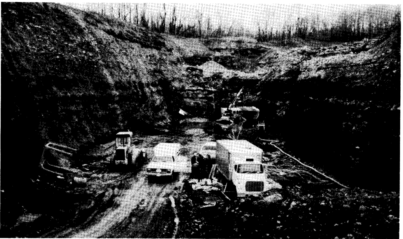
FIGURE 2. - Pit in which highwall shots were fired.
