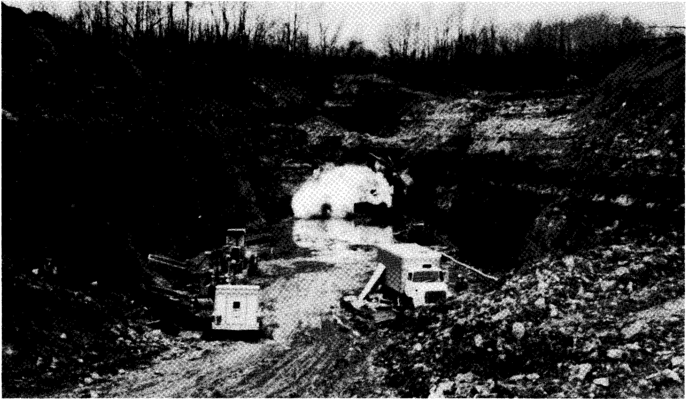
FIGURE 8. - Planned ignition of incendivity test gallery in a shot against the highwall face. Ignition was caused by loading the first hole beyond the collar without stemming.
