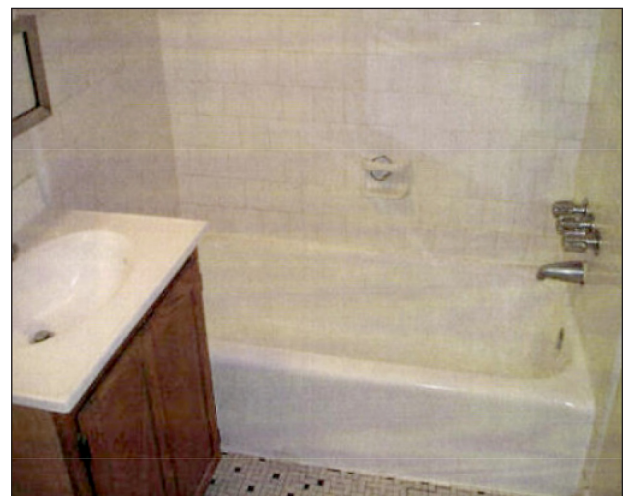
Photo courtesy of Maryland Occupational Safety and Health
