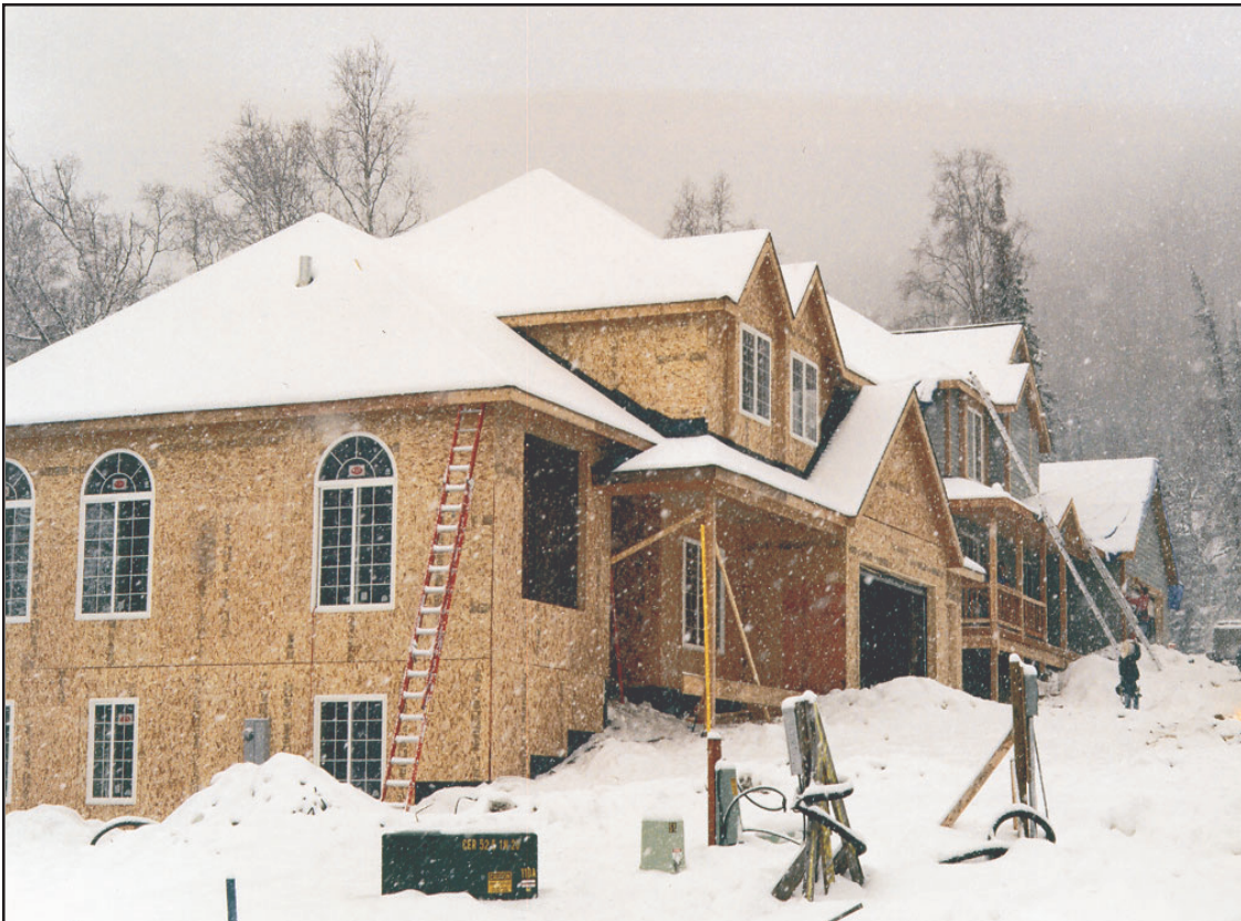
Photo 19: Residential construction site in southcentral Alaska
