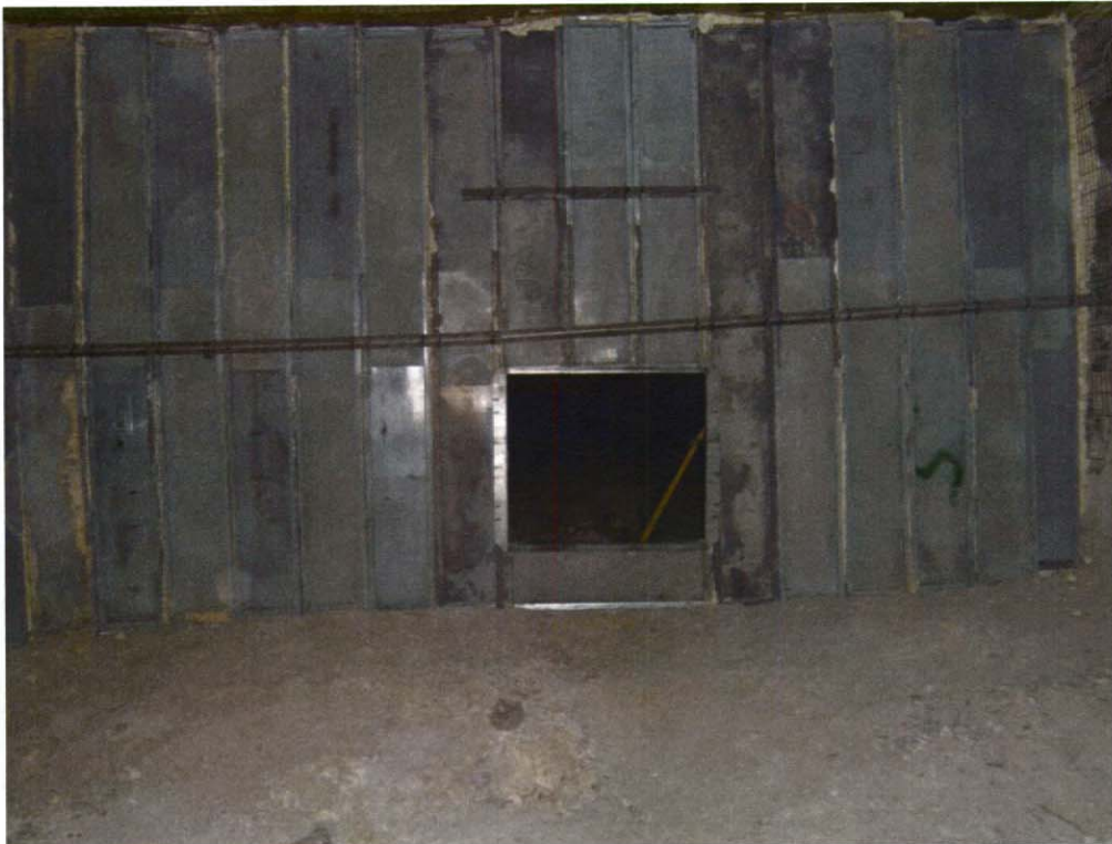
#6 Shaft Stopping (South)
