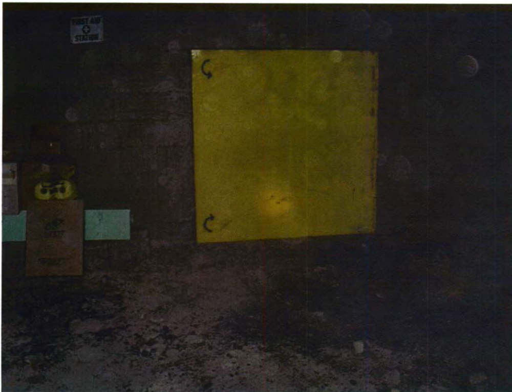
View of chamber entry door
