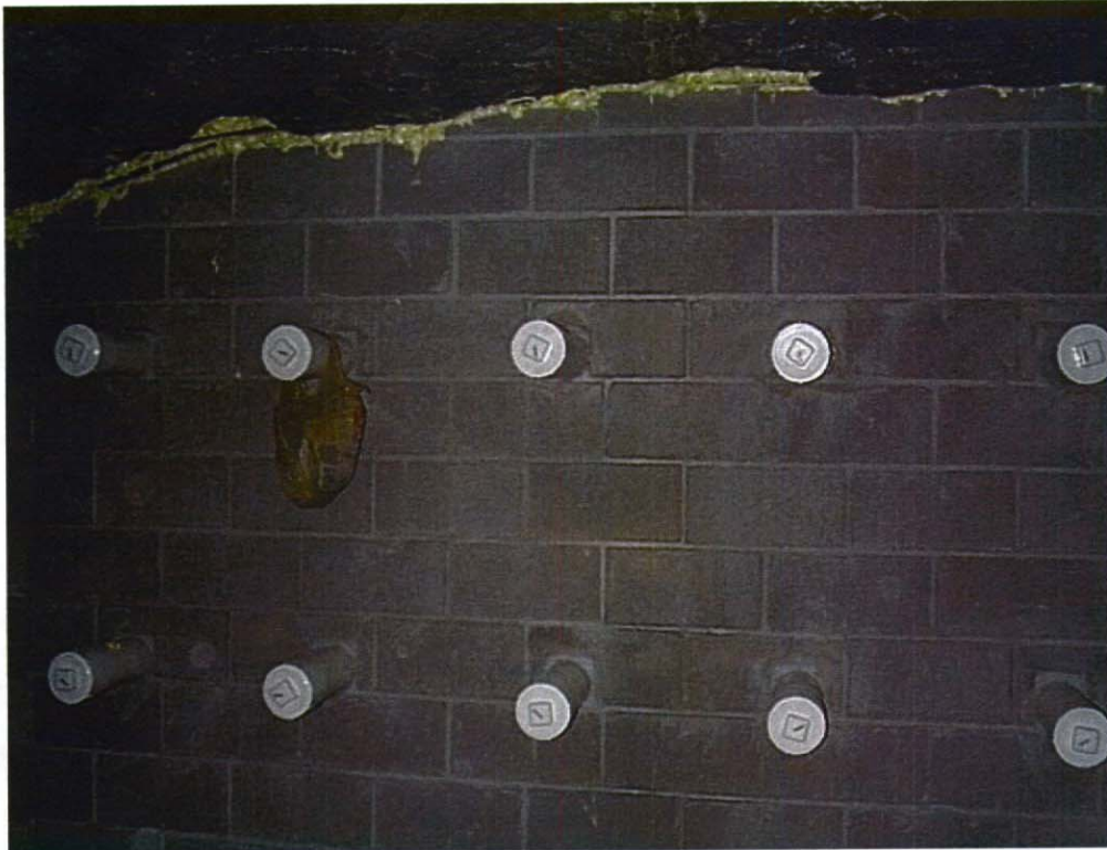
Air control pipes
