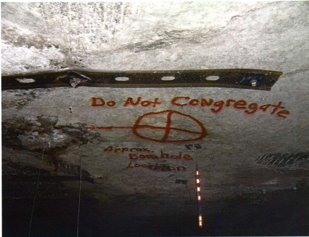
M20 Borehole location
