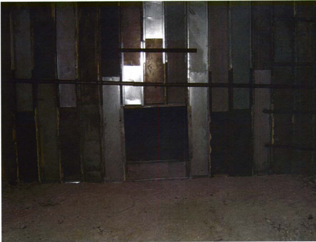
#6 Shaft Stopping (Inside)
