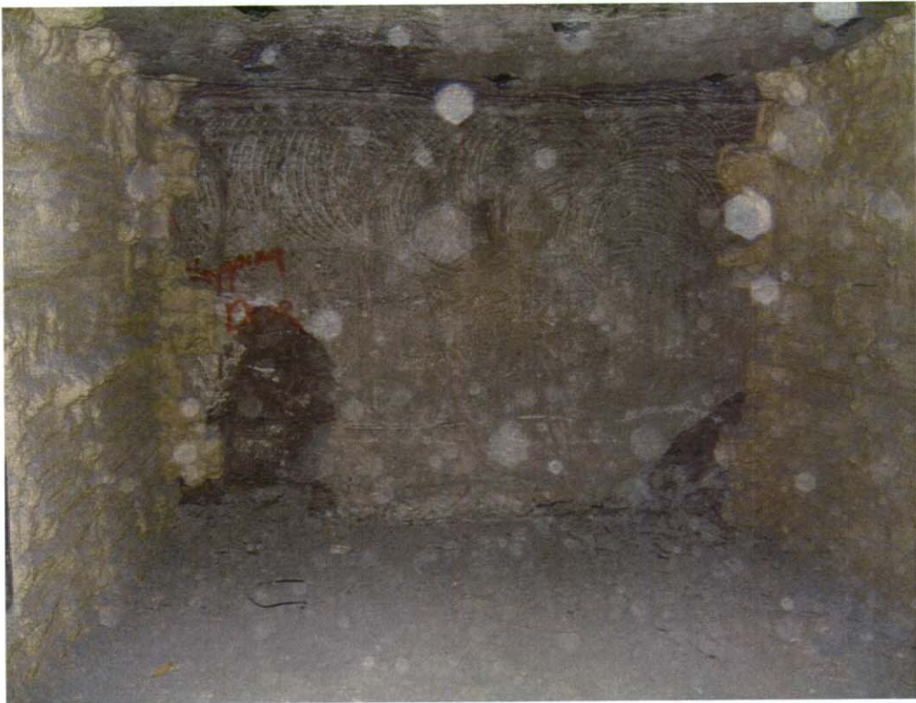
Air lock to M20
