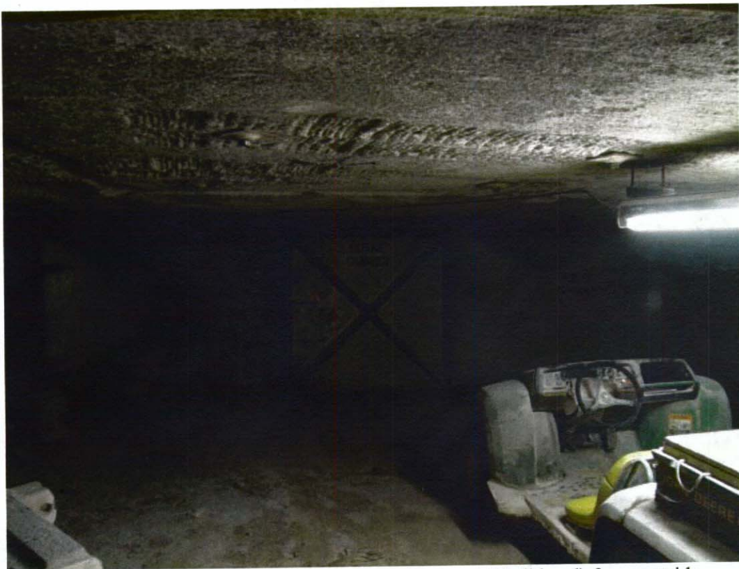
Figure 3. East Mine refuge chamber door (and metal bulkhead) from outside.
