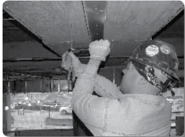
Problem: Tightening conventional nut on all-thread
