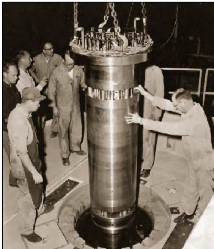
Figure 5-4: Installation of EBR-I Reactor Vessel
