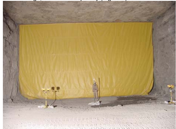
Figure 8. Tightly installed brattice stopping in a large-opening mine [16.8 m x 8.5 m (55 ft x 28 ft)]
