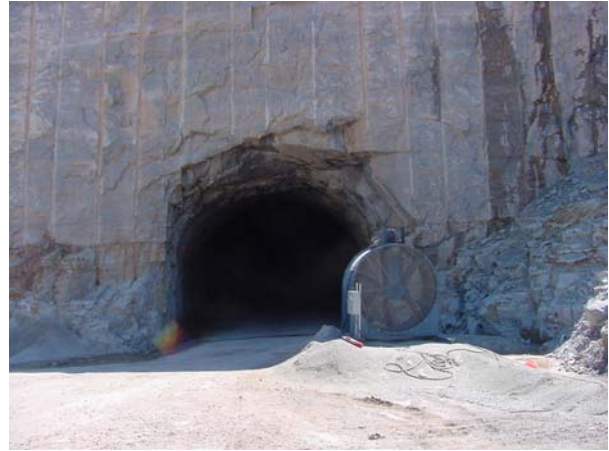
Figure 3. Propeller fan blowing into a new mine using split-mine ventilation
