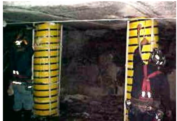
Figure 1. Pumpable roof support being installed in a longwall tailgate.
