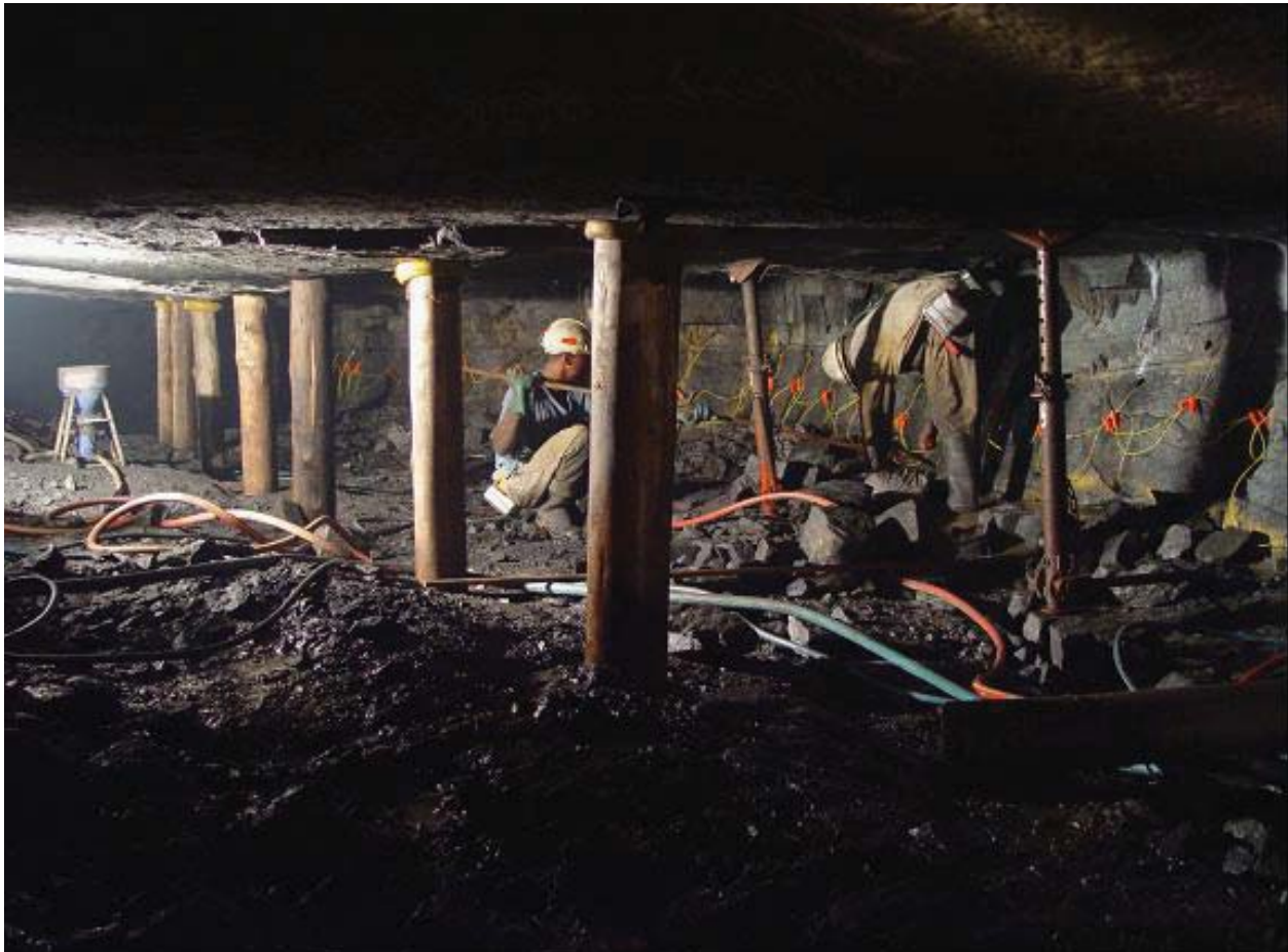
Figure 7: Prestressed props can be employed along face line as they can withstand the ground reaction and force from the blasting at the face.
