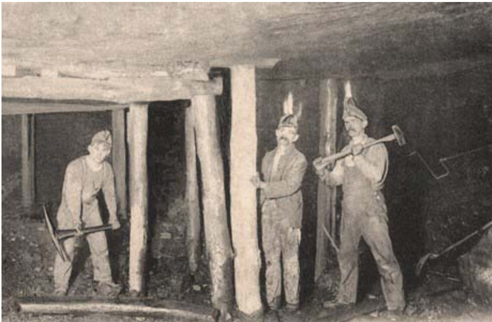
Figure 1: A historical photograph of miners setting timber posts and beams.
