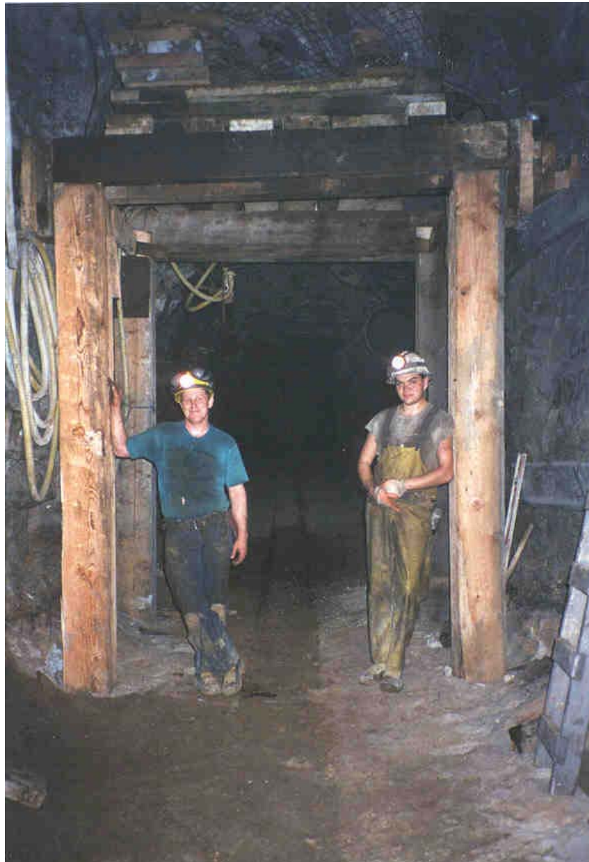
Figure 2: Traditional timber sets for hardrock applications.
