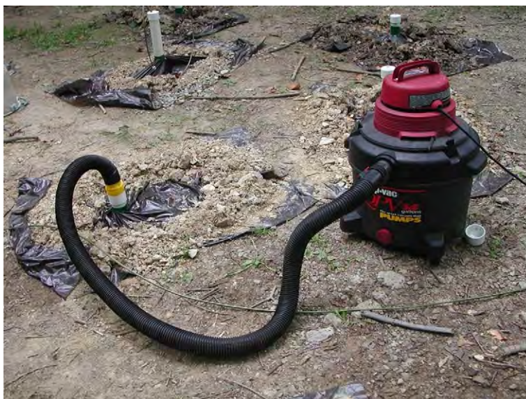
Fig. 3. Negative pressure application using a Shop-Vac.
