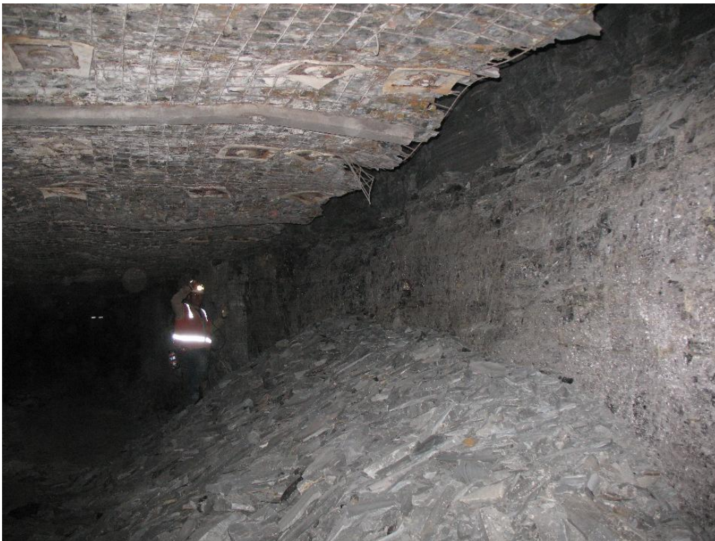
Figure 23: Rock pile below rib gutter is due to disaggregation of weak roof shale.
