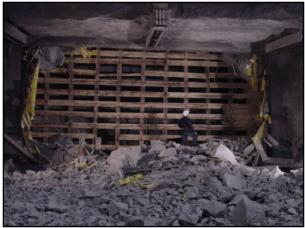
Remains of a cementitious seal after a methane air explosion.
