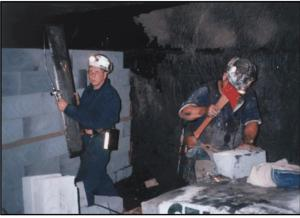
Installing load cells in a ventilation stopping in a longwall headgate to measure load development.
