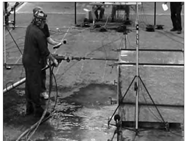
Figure 3—Drilling with the SECO S215
