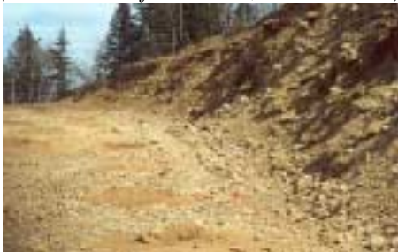
Figure 3. Minor raveling along a bench face
