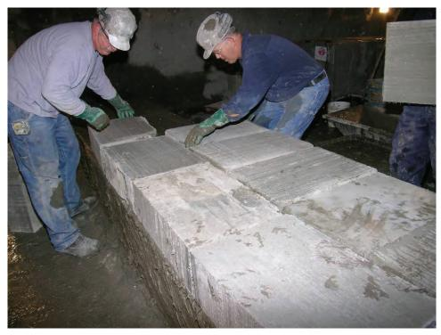
Figure B-26.—Positioning the second course of Omega blocks in a transverse pattern.
