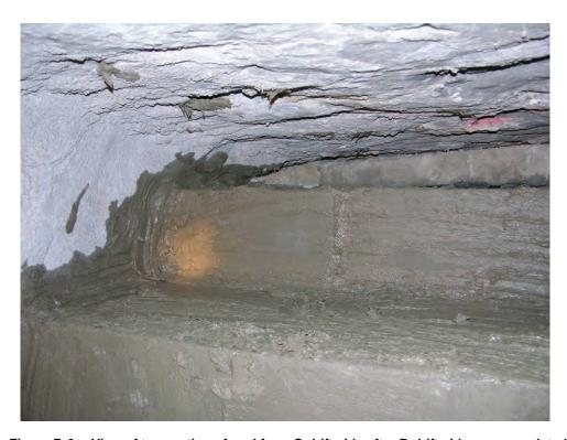
Figure B-6.—View of top portion of seal from C-drift side after B-drift side was completed. The last two block courses and middle and inby crossboards were installed from the C-drift side to complete the seal.
