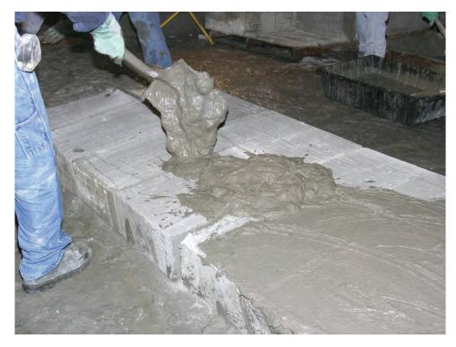
Figure B-20.—Applying the properly mixed BlocBond to the first course of Omega blocks.
