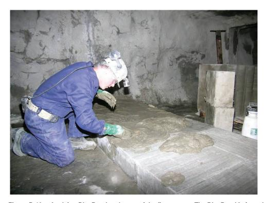
Figure B-13.—Applying BlocBond to the top of the first course. The BlocBond is forced into the vertical joints using only gloved hands.
