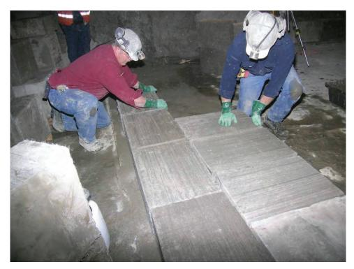
Figure B-12.—Positioning the first course of Omega blocks.
