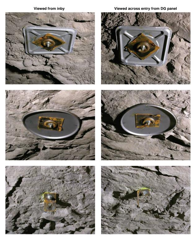
Figure 6.—Roof plates and belt hanger at 234 ft from the face.
