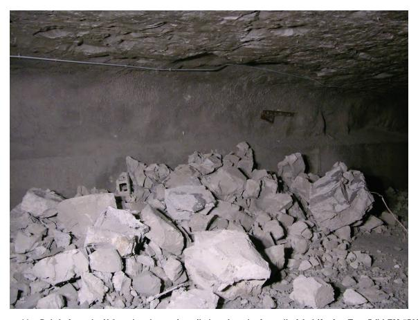
Figure 44.—Debris from the X-3 seal and stopping piled against the far wall of A-drift after Test 5 (LLEM #505).
