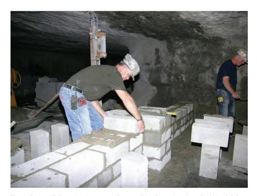
Figure B-28.—Full wet-bed construction on all horizontal and vertical block joints.
