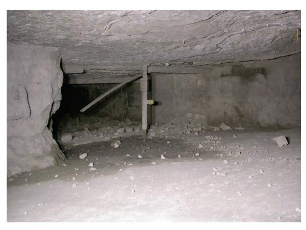
Figure 41.—Debris from X-3 seal after Test 5 (LLEM #505) viewed from C-drift.
