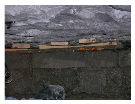
Figure B-9.—Closeup of the wood wedges, installed between the mine roof and the rough-cut board, used to tighten the Omega block seal.
