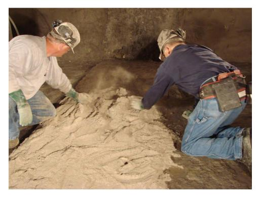
Figure B-18.—Applying the 1.5-in-thick layer of dry BlocBond to the dampened concrete floor in X-3.
