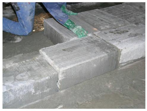
Figure B-24.—Positioning the Omega blocks in a staggered pattern for the first course.
