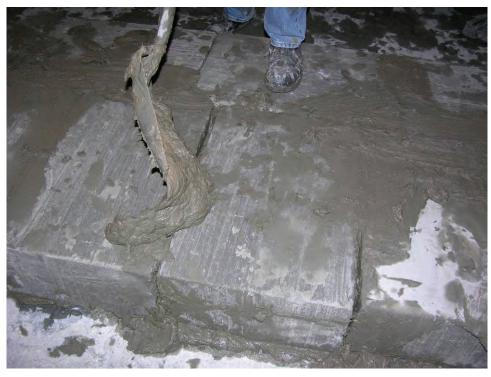
Figure B-2.—BlocBond being applied to gaps between the Omega blocks.
