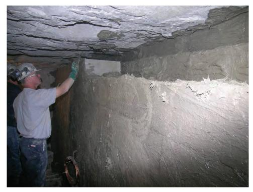
Figure B-16.—Completing the 11th and final full block course on the outby side.
