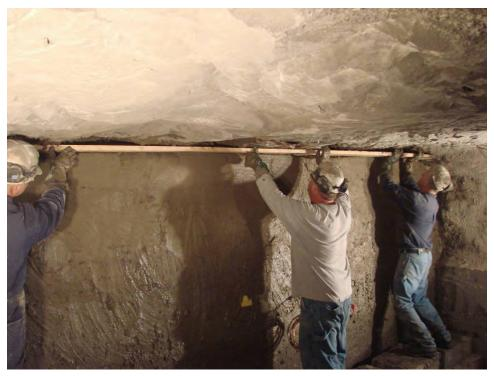
Figure B-27.—Installing the crossboard on the outby side of C-drift seal.
