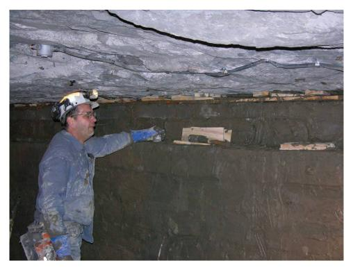
Figure B-8.—View from the C-drift side showing the rough-cut lumber wedged between the mine roof and blocks across the center of the seal.
