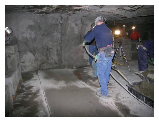
Figure B-11.—Wetting the dry layer of BlocBond before positioning the Omega blocks.
