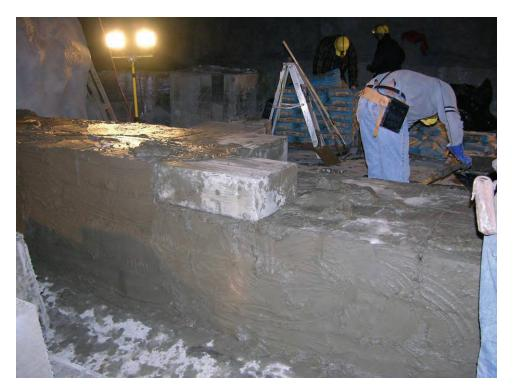
Figure B-3.—As each Omega block course was completed, BlocBond was also coated on the exposed B- and C-drift sides of the blocks.
