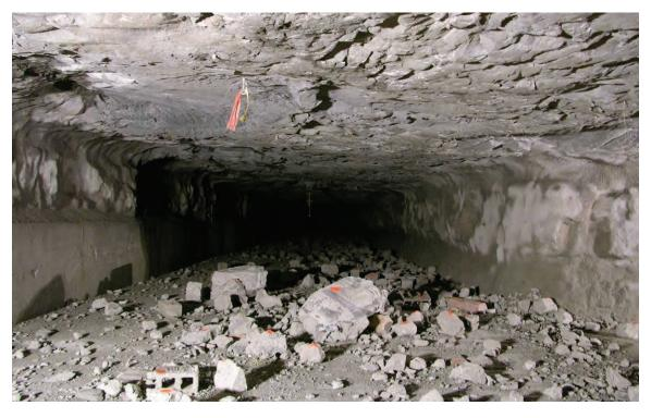
Figure 48.—Debris in C-drift after Test 5 (LLEM #505) looking outby from X-6 at 547 ft.
