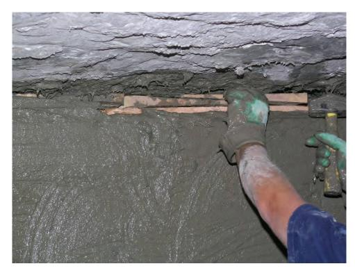
Figure B-21.—Driving the wedges (skin to skin) between the crossboard and mine roof.
