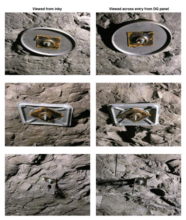
Figure 5.—Roof plates and belt hanger at 134 ft from the face.
