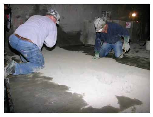
Figure B-22.—Applying a 1.5-in-thick layer of dry BlocBond on the dampened concrete floor across C-drift.
