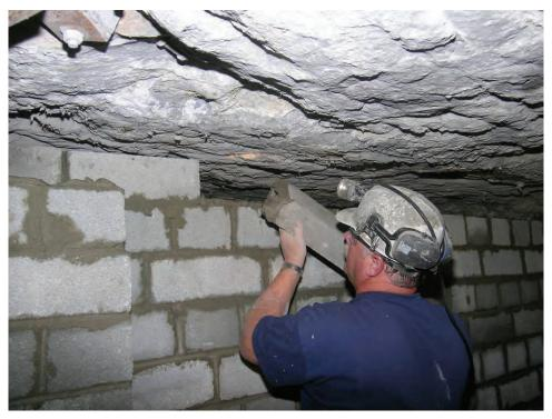
Figure B-29.—Installing cut blocks on top course.
