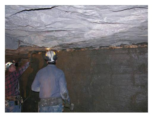
Figure B-7.—One row of wood placed flush with the edge of the blocks on the B-drift side.
