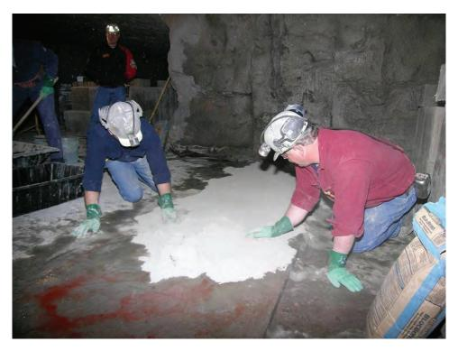
Figure B-10.—Dry BlocBond being spread to a 0.5-in-thick layer on the dampened concrete floor in X-3.
