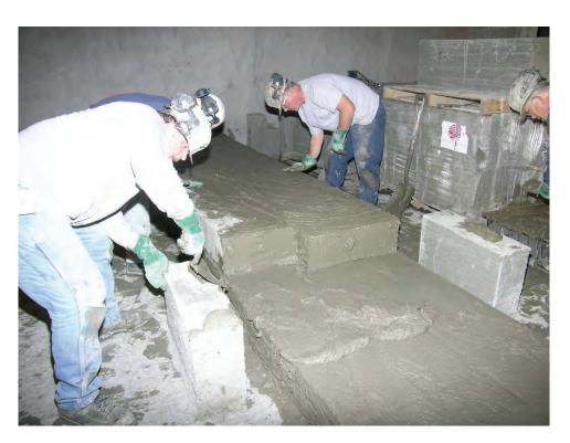
Figure B-15.—Omega blocks laid wet with fully mortared (BlocBond) horizontal and vertical joints.
