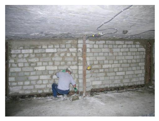
Figure B-31.—Mortar filling the gaps between the steel angle hitching and the blocks along the floor and ribs.
