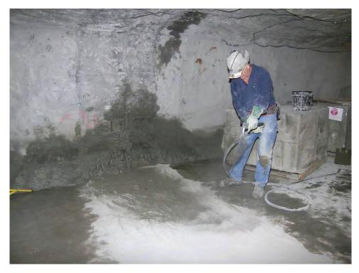
Figure B-23.—Wetting the dry layer of BlocBond with a fine spray of water.
