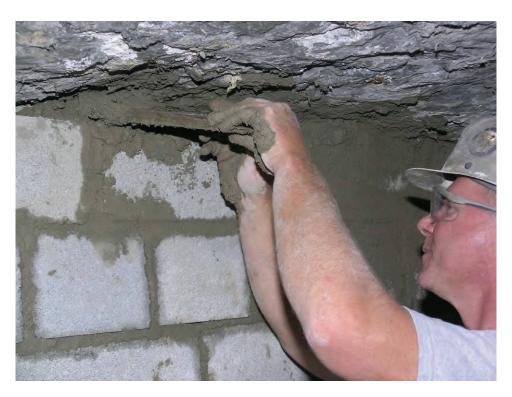
Figure B-30.—Completely filling the gap between the top course of blocks and the mine roof with mortar. The blocks were not wedged.
