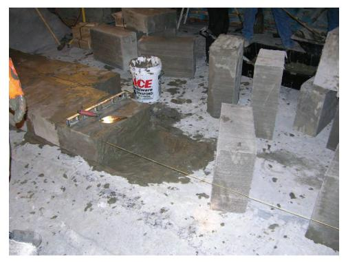
Figure B-1.—BlocBond applied to concrete mine floor.
