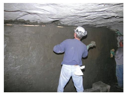
Figure B-17.—Hand slinging the BlocBond to fill the gaps between the previously installed center board and the outby board.
