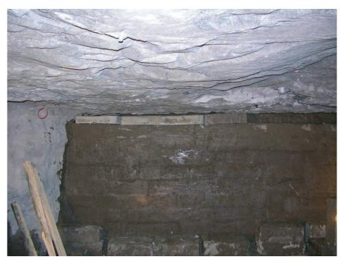
Figure B-5.—Cut blocks on top course to provide 2-in gap to roof.
