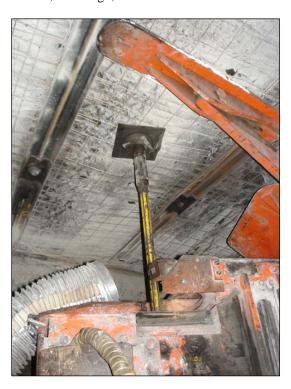
Figure 4.—Once drilling is completed, the CDSE is moved aside so the roof bolt can be installed.
