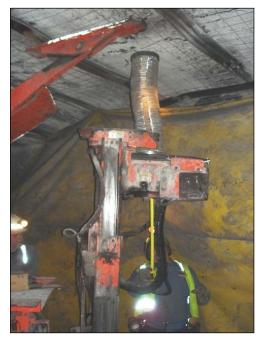
Figure 3.—As drilling advances, the CDSE collapses.
