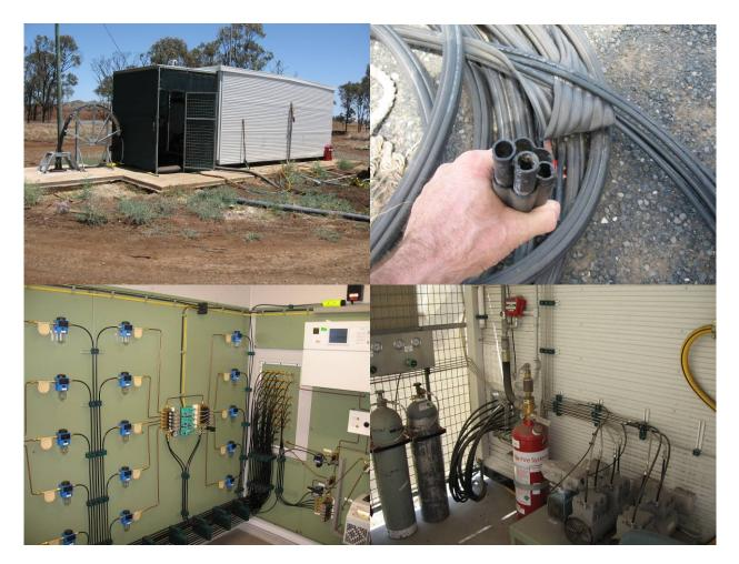
Figure 8.—Continuous atmospheric gas monitoring system in Australia. *Top left:* Monitoring shed over mine showing borehole and sample tubes. *Top right:* Close-up of sample tube bundle. *Bottom right:* Sample tube pumps. *Bottom left:* Inside monitoring shed showing manifold and gas analyzer.
