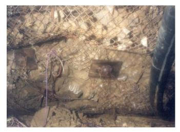
Figure 18.—Backfill failure at four-way bracket.
