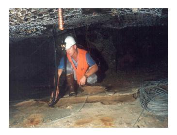
Figure 9.—Thrust-fault-type failure, November 4, 1997.
