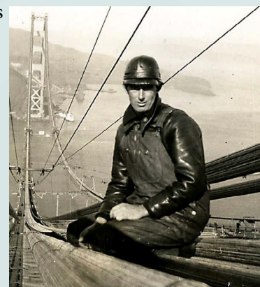
A Golden Gate construction worker wears a Bullard “Hard Boiled Hat” in this photograph, circa 1936. Credit: Labor Archives and Research Center, J. Paul Leonard Library, San Francisco State University
