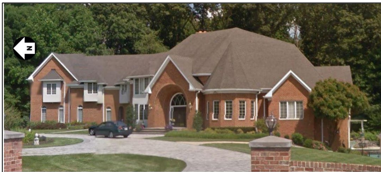
Photo 1. The 8,413 square foot custom-built home showing Side Alpha. (Photo courtesy of the Fire and Rescue Department.)
