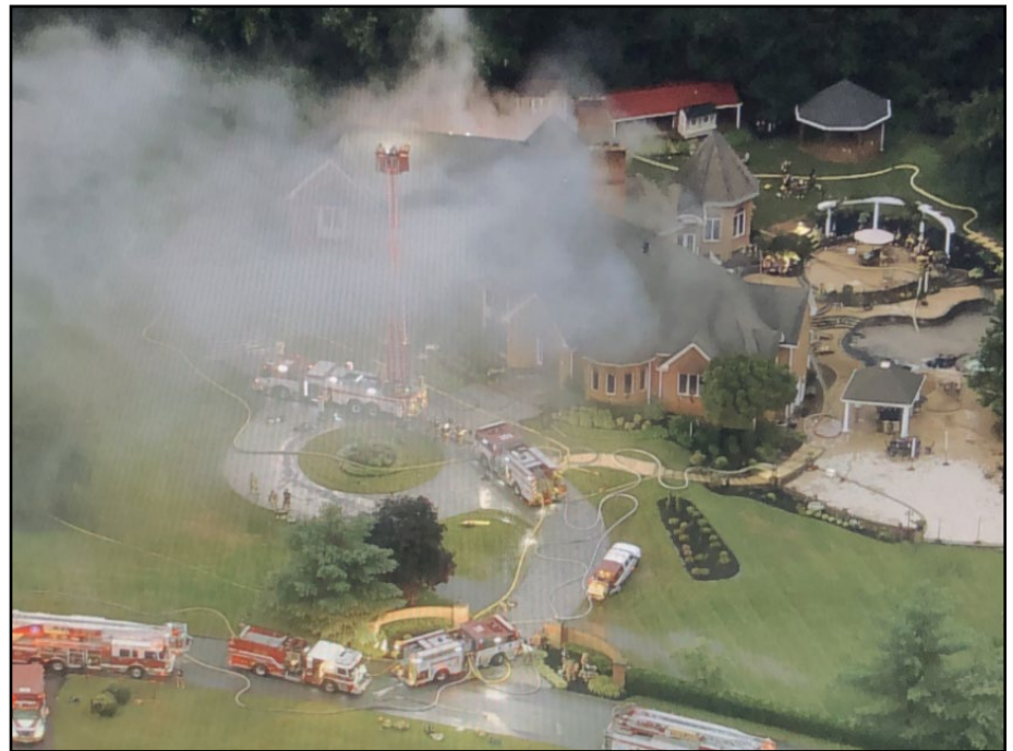
Crews operating in a defensive strategy working to knock down the fire in 8,400 square foot single-family home. (Photo courtesy of the Fire and Rescue Department)
