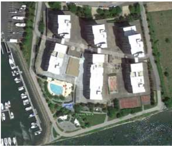
Figure 1 – Overhead view of condominium complex.
