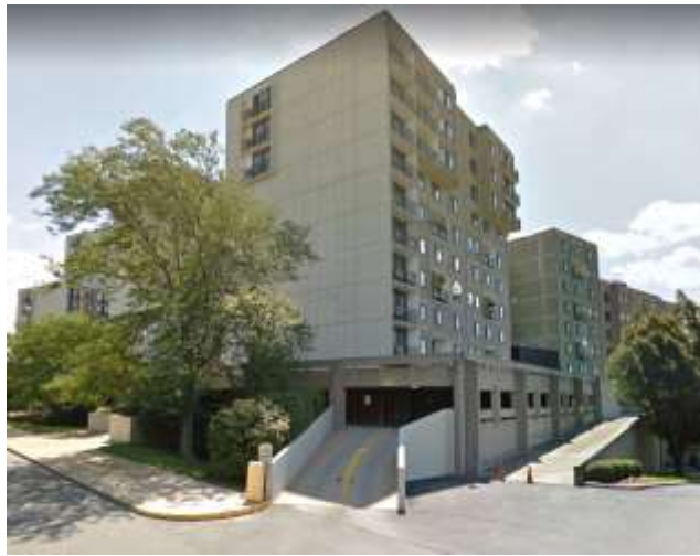
Figure 2- Outside view of residential structure with parking garage below.
