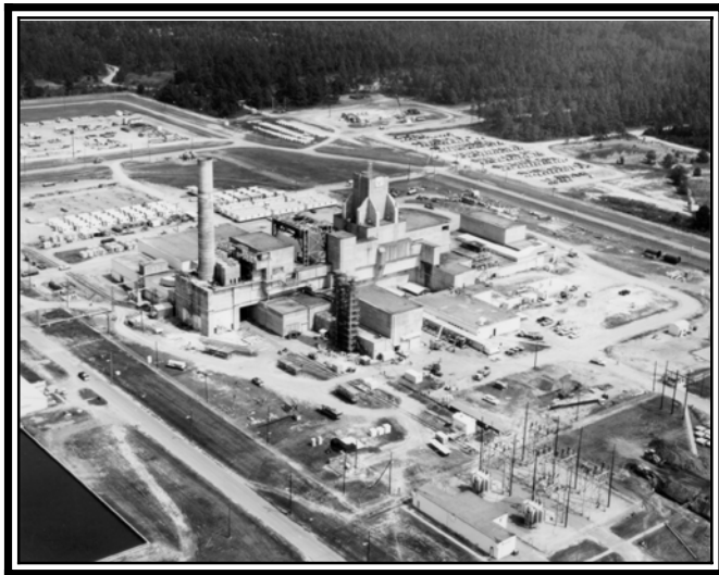
L-Reactor Facility. L Area, Savannah River Site, South Carolina. September 16, 1982. Photo courtesy of the U.S. Department of Energy.
