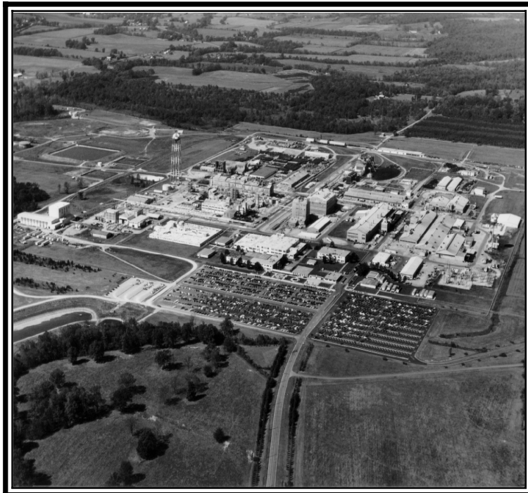
Feed materials Productions Center (FMPC). Fernald , 20 miles outside Cincinnati, Ohio. January 1, 1987. Photo courtesy of the U.S. Department of Energy.
