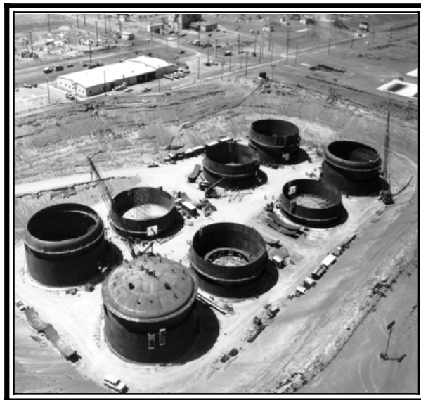
Storage tanks for high-level liquid radioactive waste at Hanford. Hanford Site, Richland, Washington. October 31, 1984. Photo courtesy of the U.S. Department of Energy
