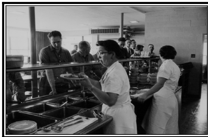
Cafeteria. Idaho National Engineering and Environmental Laboratory, Idaho Falls, Idaho. 1957. Photo courtesy of the U.S. Department of Energy.
