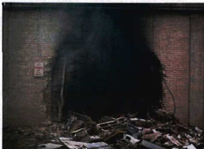
The "punch out" hole in A-E Drive.
