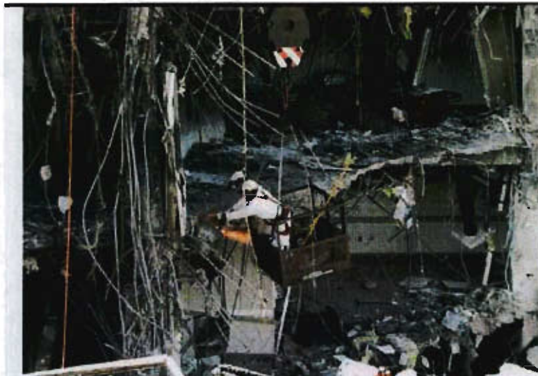
Demolition in preparation for reconstruction.
