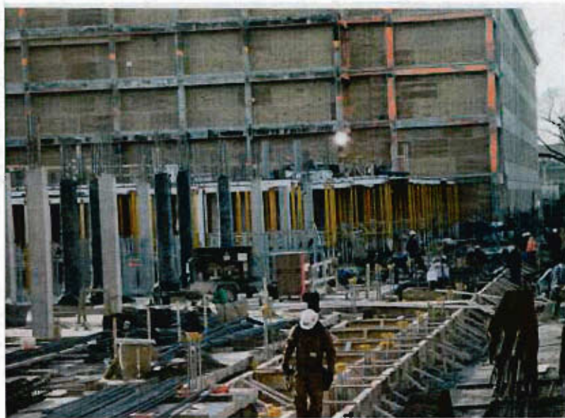
Reconstructing the damaged area.
