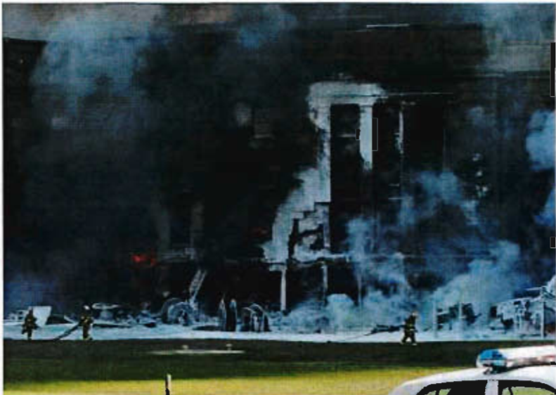
Foam residue visible on the Pentagon facade, before the collapse.
