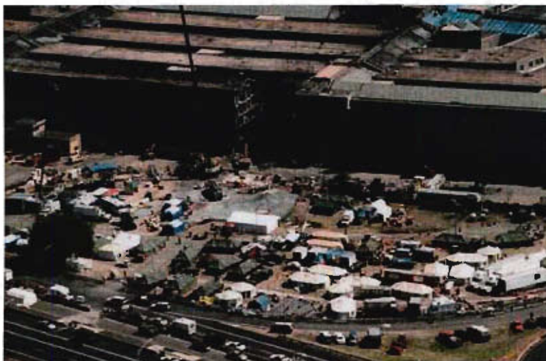
Days after the attack, the lawn west of the Pentagon filled with vehicles, equipment, and tents for command and control, search and recovery, shoring, demolition, and security.
