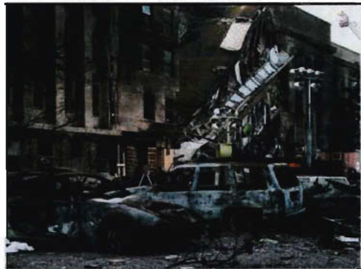
Heliport air tower controllers' burnt cars.
