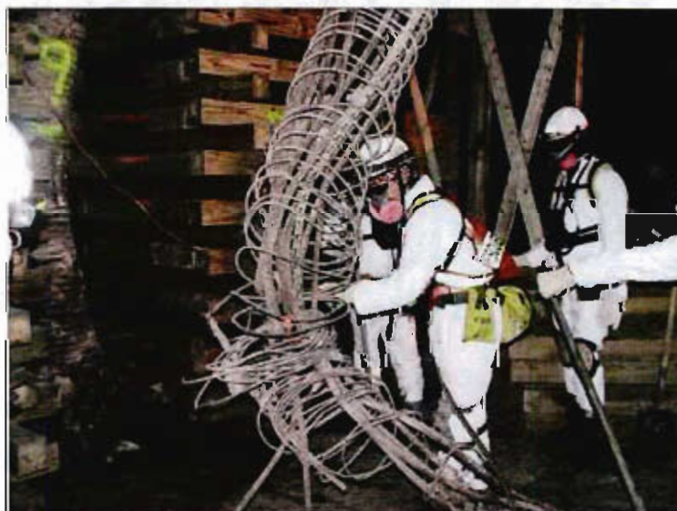
Removing a damaged building column.
