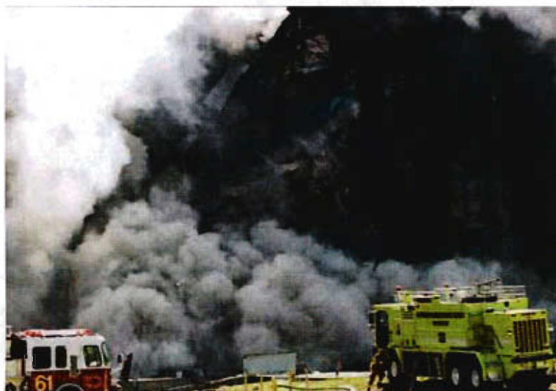
Firefighters pull back as part of the E Ring collapses.
