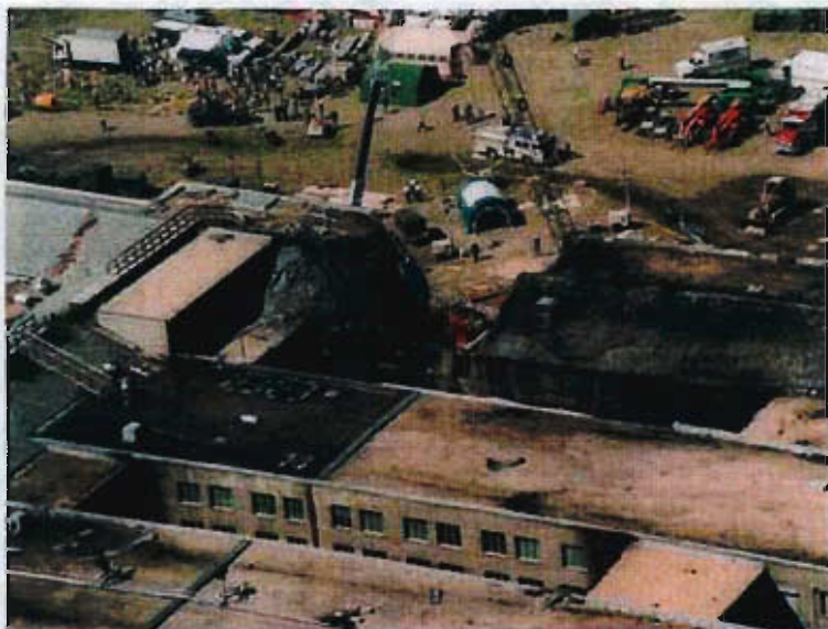
The inner E Ring wall still stands days after the collapse.
