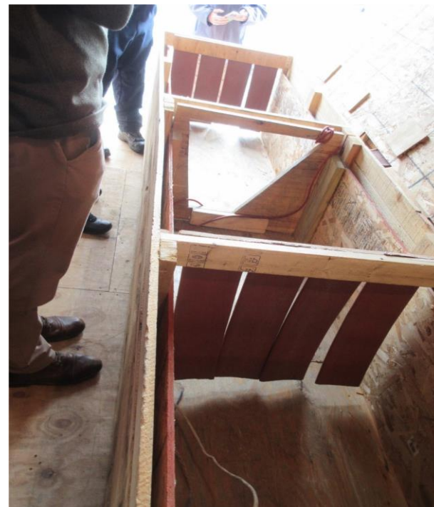
The third restricted opening in the tunnel prop (Photo by NIOSH)
