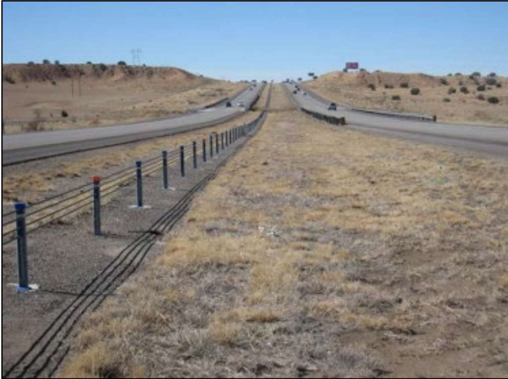
Incident site looking south; note gentle down-slope to north end of bridge. (NIOSH photograph)
