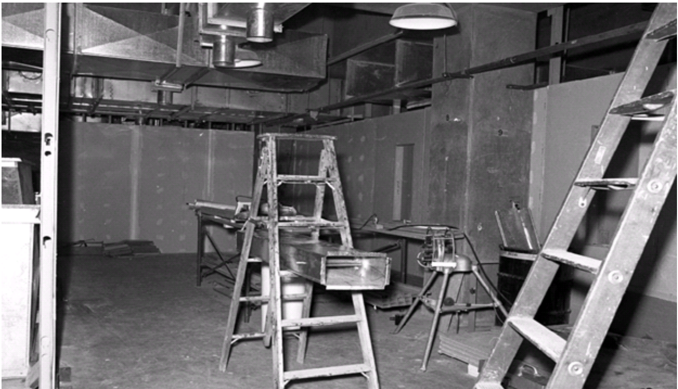
Figure E-7. Construction of a support room, February 26, 1975 (DuPont 1975i) (DPSPF 18813-28).
