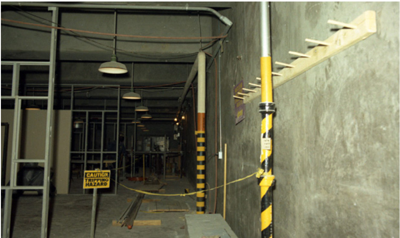
Figure E-10. Room construction demonstrating safety awareness and hazard markings, November 20, 1976 (DuPont 1976i) (DPSPF 18678-24).
