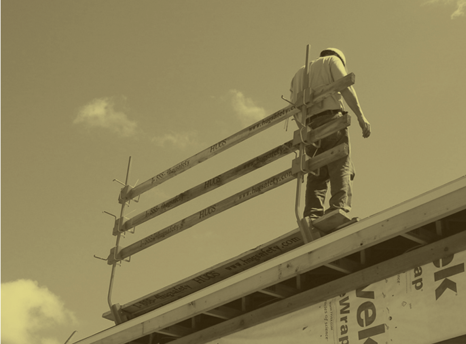
A construction worker leans against the guardrail during a field trial of the Adjustable Guardrail Bracket. The unit is attached to a sloped residential roof. Photo by Thomas G. Bobick
